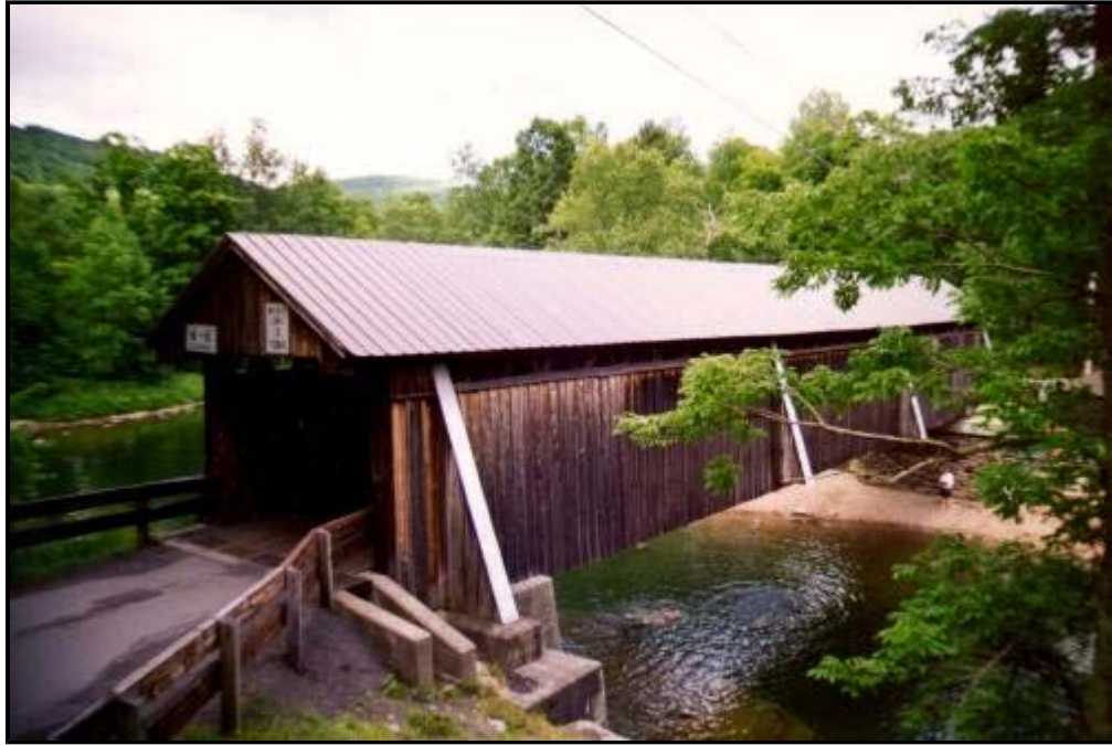
Beaverkill bridge in the summer
