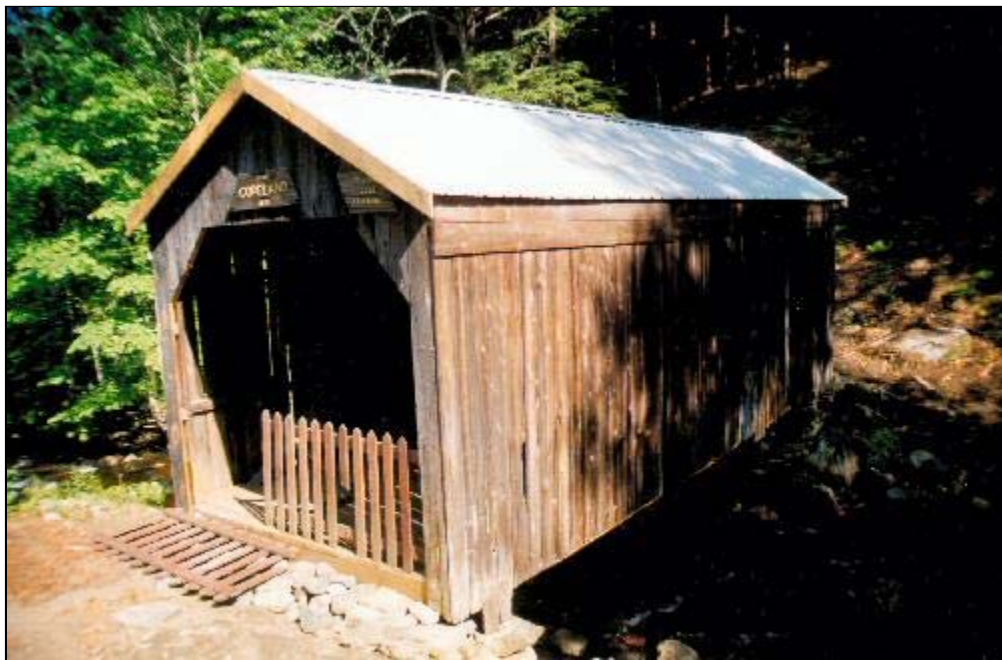
Copland Bridge Portal Photos
