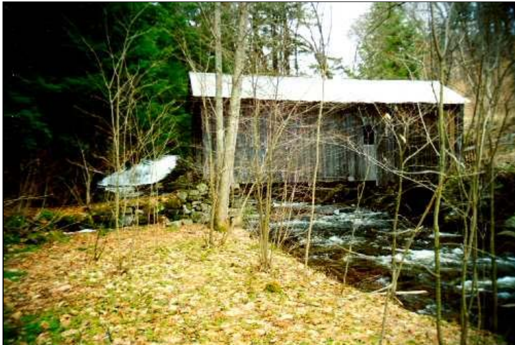
Copeland Bridge in the Winter and Fall
