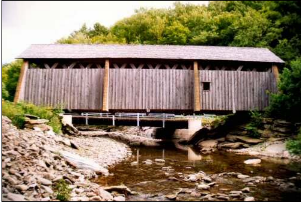
Photo of Grants Mills Bridge
