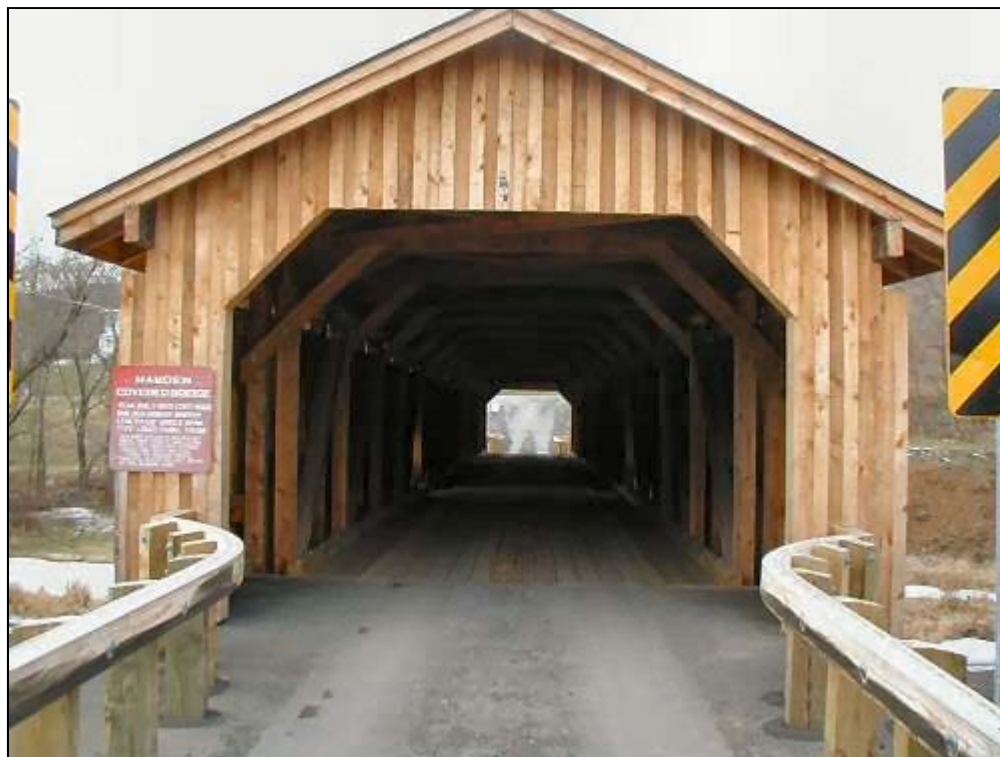
Hamden Bridge Portal - January 5, 2002
