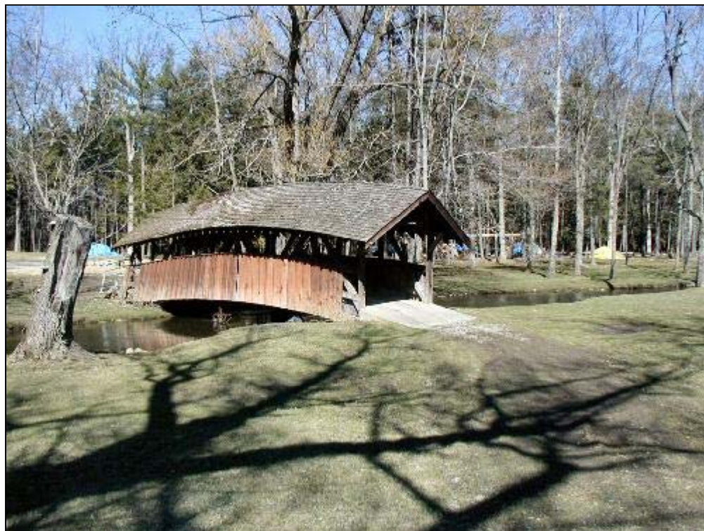
Photo of Mead Bridge
