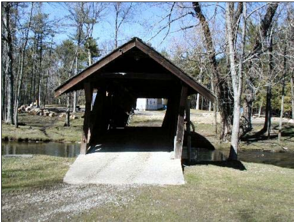
Photo of Mead Bridge Portal
