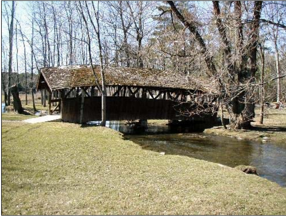
Photo of Mead Bridge
