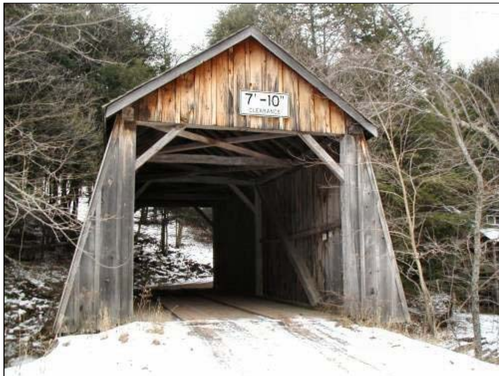
Tappan Bridge Portal
