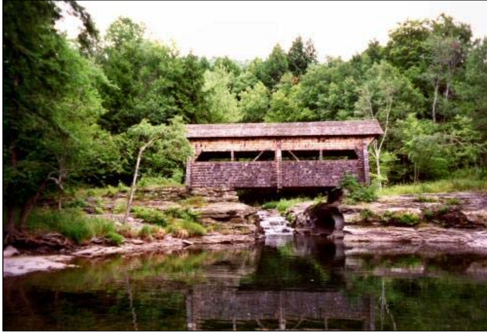
Photo of Tuscarora Club Bridge
