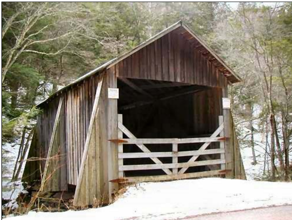
Forge Bridge Portal
