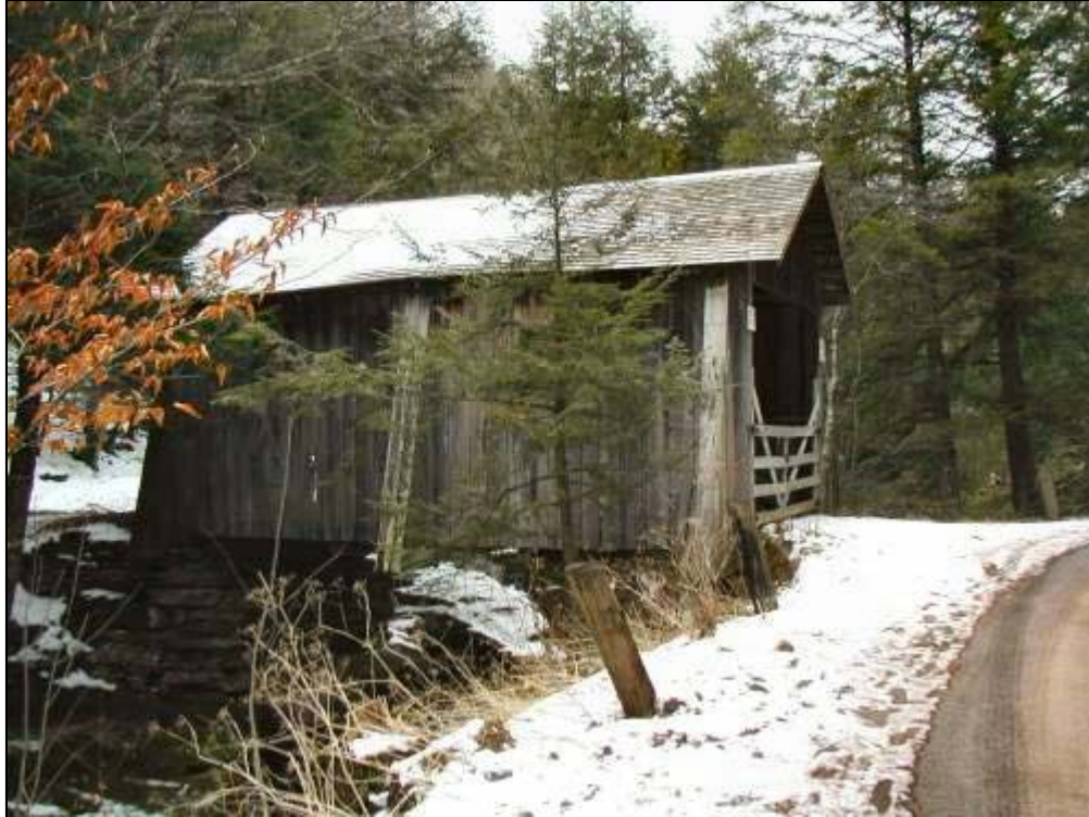
Photo of Forge Bridge
