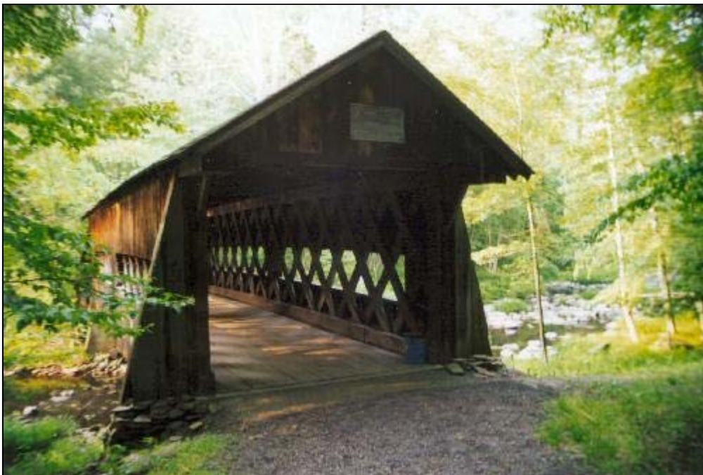
New Paltz Campus Bridge Portal
